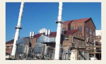
At Sainte-Emilie, a large investment of 25 million euros, including 6.9 million in State subsidies, has been spent on a new indirect sugar beet pulp dehydration unit which will be operational in September 2023. This will enable residual heat from the plant to be recovered and will in turn end the use of coal. A 90% reduction is expected in  $CO_2$  emissions from drying. Ending the use of coal will also lead to a reduction in the quantity of particulate matter and sulfur being produced.
