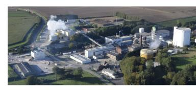
In 2019, the Fontaine-le-Dun site started up its new methanation unit supplied with water from the sugar refinery. Operational during the last two sugar beet campaigns, the device has generated biogas and currently supplies 7% of the sugar refinery boiler requirements.
